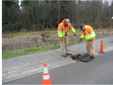
Catch Basin Inspection and Cleaning
