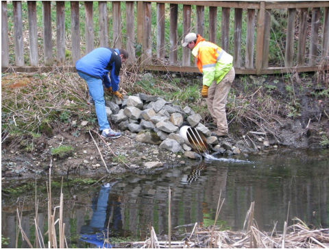
Storm Pond Inspection and Maintenance
