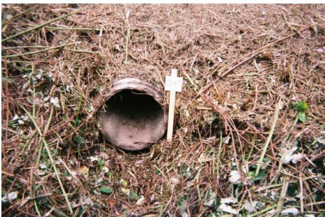
Outfall and Receiving Water Survey
