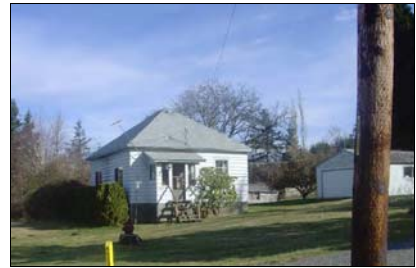
House at 26209 Lawson Street
